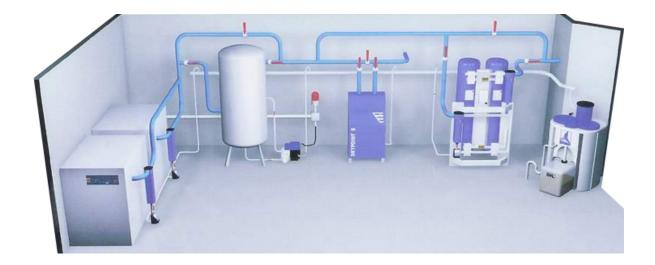
**FRL-units** are an important element of the pneumatic system. With these units the air can reach the required quality since they have filters for cleanness, lubrication for oil content and can manage pressure. Well-processed air does not only ensure a safer workspace but also increases the durability of the equipment.
